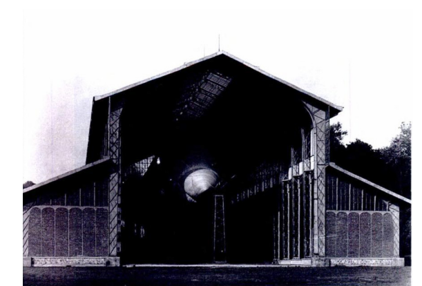
Figure 3 The hangar used by Renard and Krebs with steel components designed by Eiffel.
